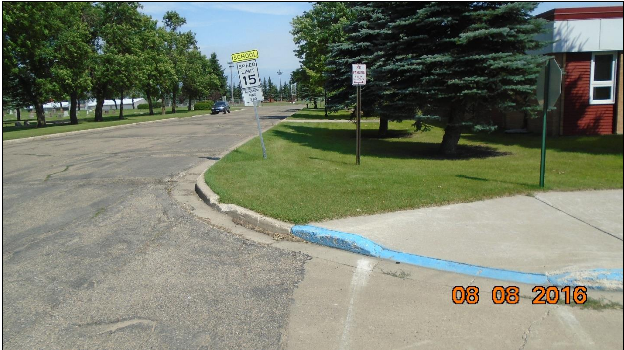
Figure 2. No sidewalk on the west side of high school
