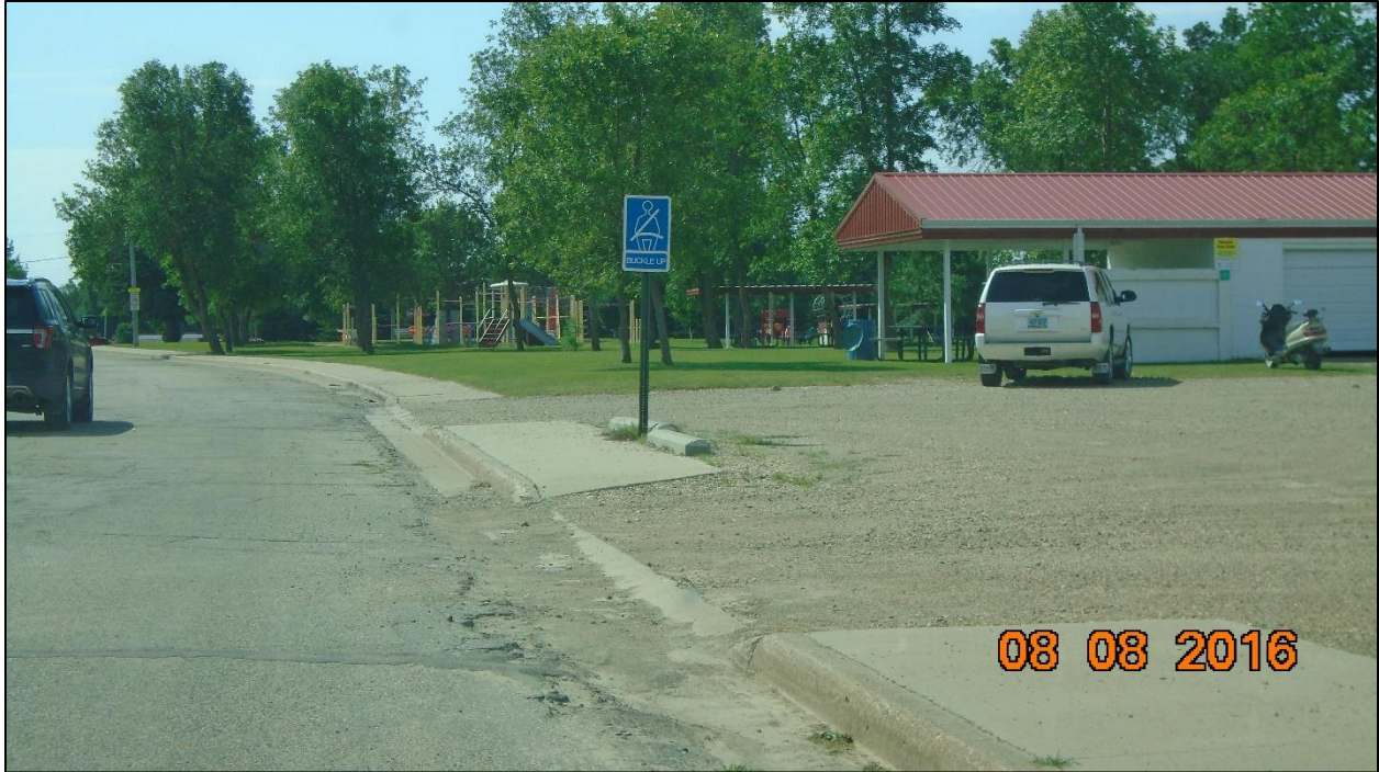
Figure 8. Sidewalk started and stopped across driveways leading to the parking lot south of high school
