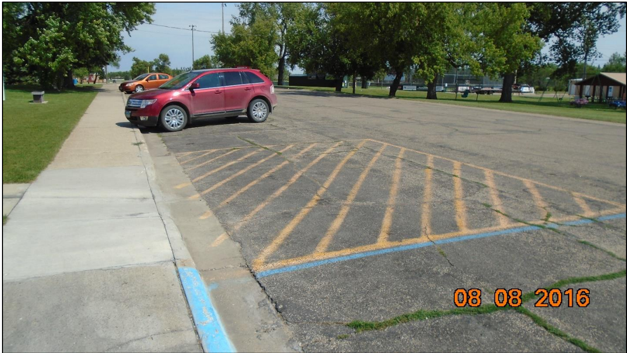
Figure 9. Ramp leading to a no parking zone on the west side of the park.
