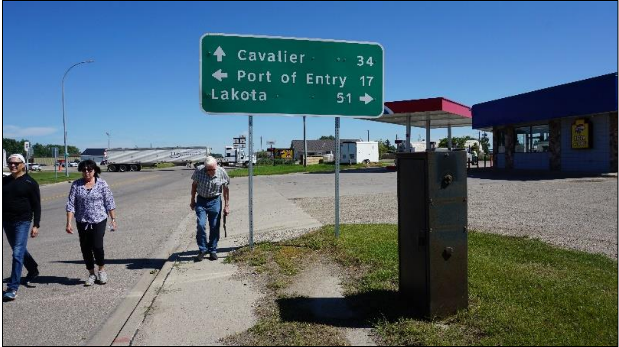
Figure 16. Guide sign obstructing the sidewalk
