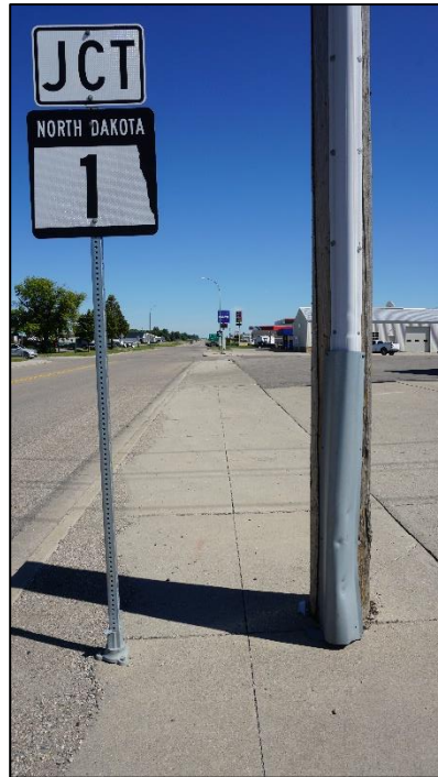
Figure 17. Route sign and utility pole obstructing sidewalk
