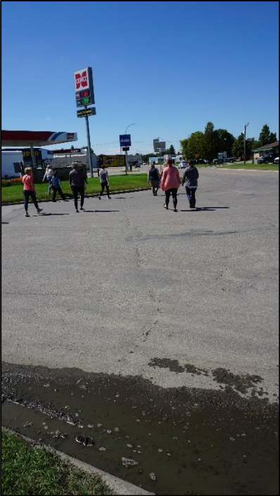
Figure 14. Lack of crosswalk/sidewalk on the south side of ND Highway 5 at ND Highway 1
